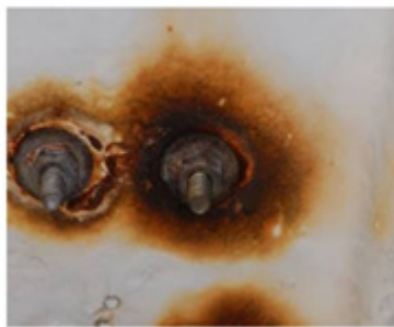
Crevice corrosion under the nuts due to the gaskets
